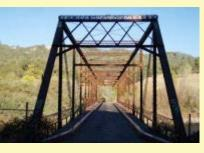
the Pratt Truss bridge links Gwin Mine Road in Calaveras County and Middle Bar Road in Amador County. The bridge¹s steel was originally fabricated in 1901. First made of timber, the bridge�s deck was replaced in 1969 with corrugated metal planking filled with bituminous pavement.
